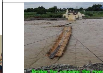
Bridge for crossing the river
